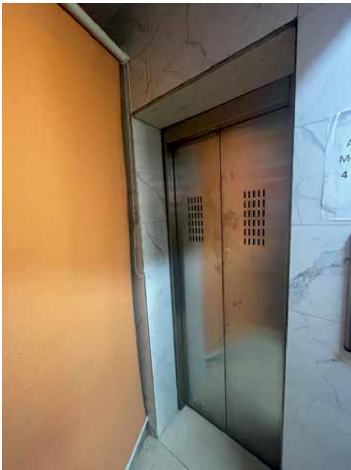
Old elevators are being replaced.
