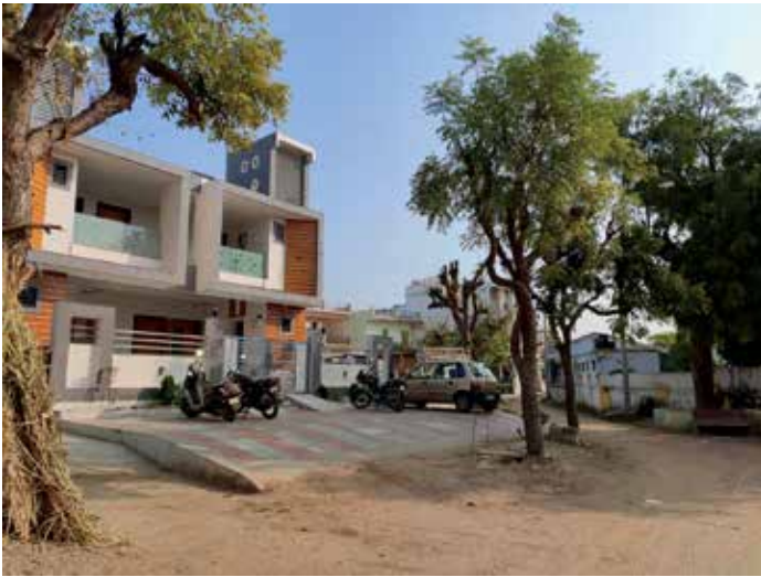
Old, small residence in Gujarat
